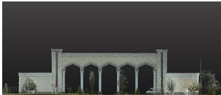
Figure 5. Rear Facade of the Building Created Based on 3D Scanning.
